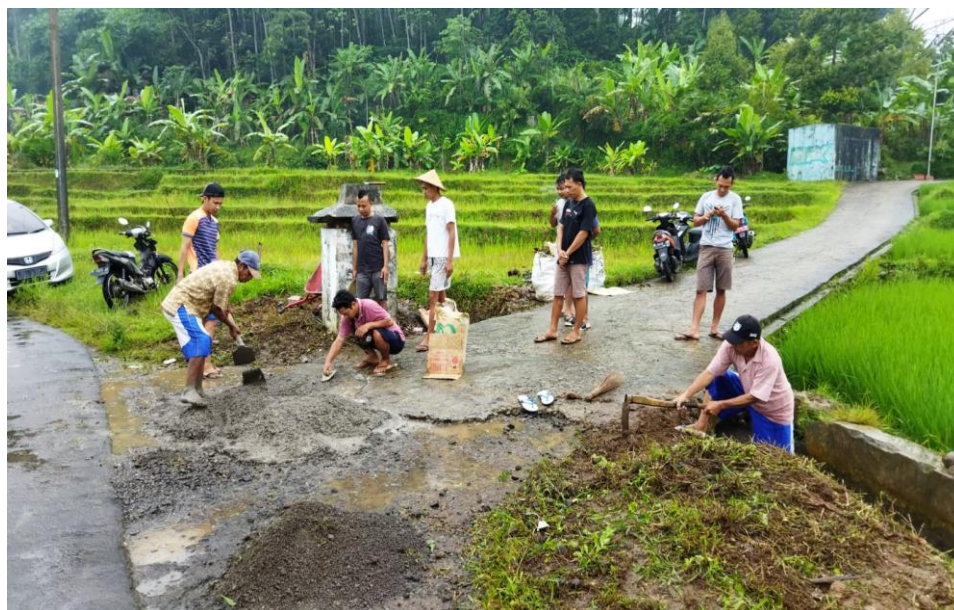
Figure. 2 Construction of cooperation of Sigaluh residents Source: documentation from researchers
